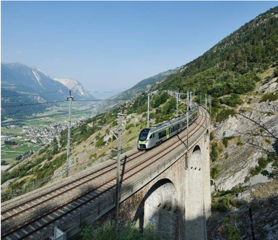
Regio Express Lötschberger, Luogelkin Viaduct near Hochtenn, Valais
